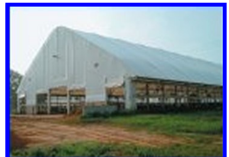
“We were able to design the barn to get all the natural ventilation we need.” says Tim Hood.
